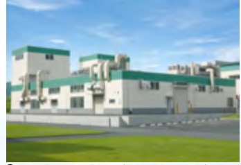
● Mie Powder Plant (Raw Materials)
